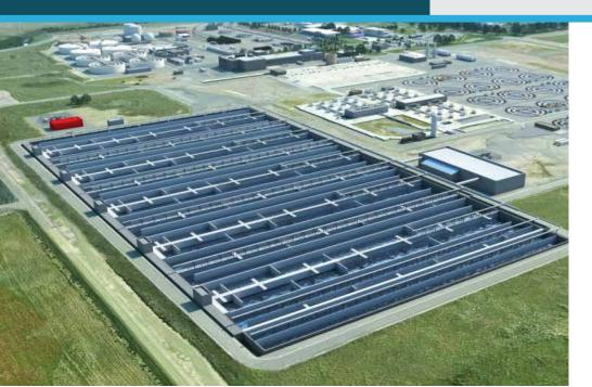
At left is an artist's rendering of the future "biological nutrient removal" (BNR) facility. This process will eliminate nearly all ammonia and most nitrate from the treated effluent. This is only one of the many new processes and facilities included in the EchoWater Project. The BNR project alone is massive – the size of approximately 20 football fields – and will cost approximately \$600 million to complete, with additional ongoing maintenance costs.
