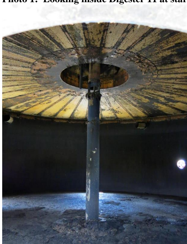
Photo 2: Looking inside Digester 11 at start of cleaning.
