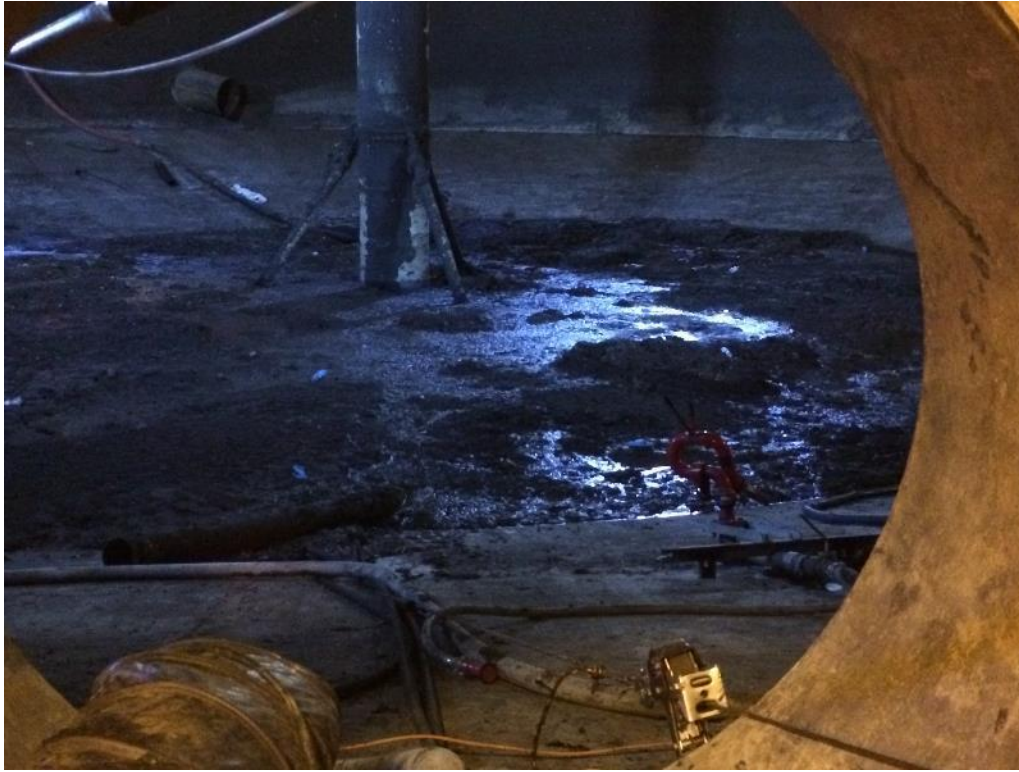
Photo 5: Looking inside Digester 11 below elevation 100ft.
