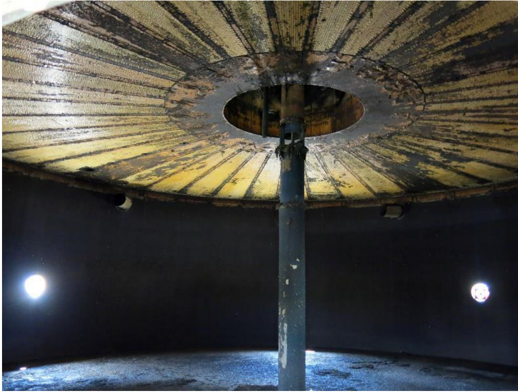
Photo 3: Looking inside Digester 11 at start of cleaning.
