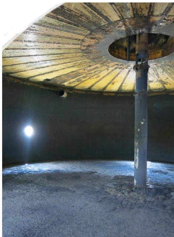
Photo 1: Looking inside Digester 11 at start of cleaning.
