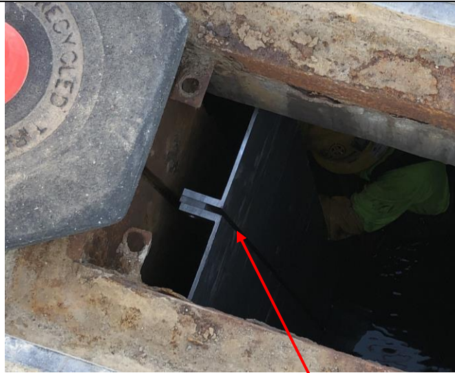
The PE gate slides in this notch.
