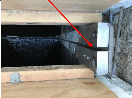
The PI slide gate slides in this notch
