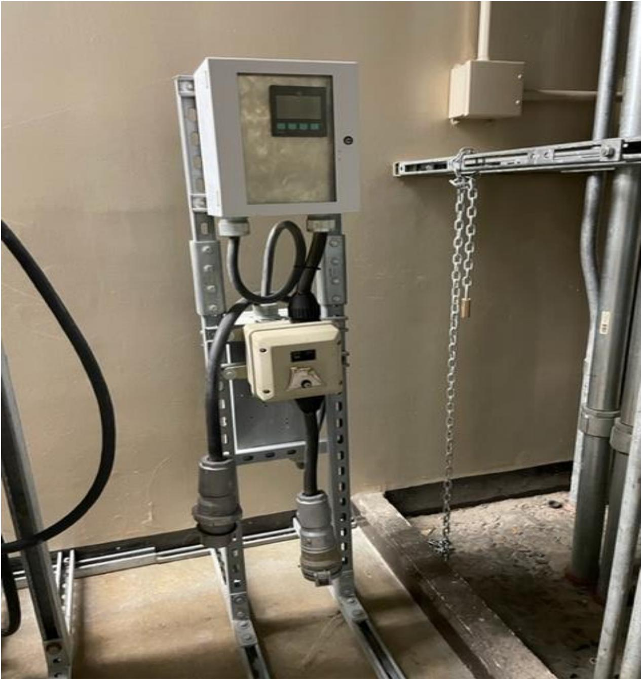
**Photo A** – 480V GFI that will be connected to field welding receptacles
