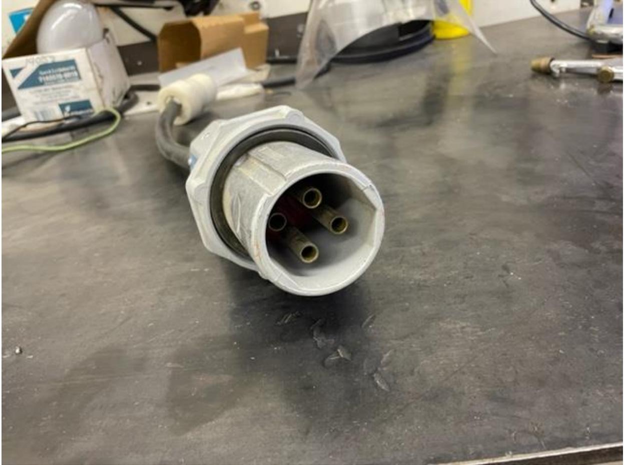
**Photo C** – 480V male connector to the GFI
