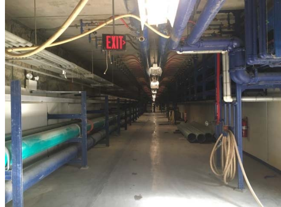
Figure 3 Existing Tunnel Section View inside Central Tunnel
